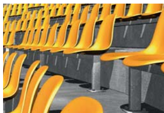
Stadium seating anchor
